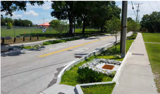
Scott Street Low Impact Development Streetscape Tampa, Florida (10/2015-04/2017)
