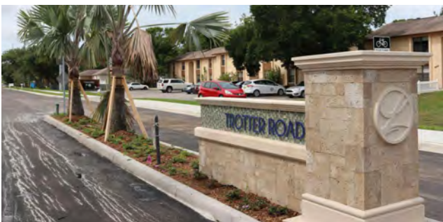
Trotter Road Streetscape Largo, Florida (03/2016-08/2018)
